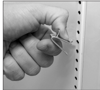
Fig. 1. Installing top tab of shelf clip.
