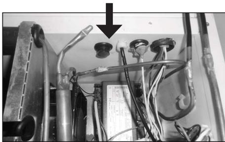
4. Inside the port hole is located in the top right side and is closed with a rubber plug.
